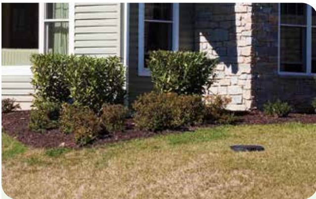
Propane storage can be buried underground with only an inconspicuous service dome showing.
